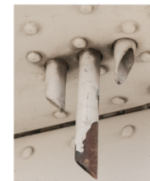
Battery Vents & Batter Drains
